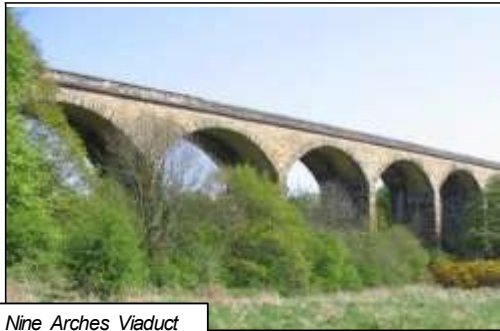
Nine Arches Viaduct
