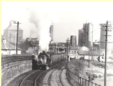
The Derwenthaugh Coke Works and the rail line along the route of the New Western Way
